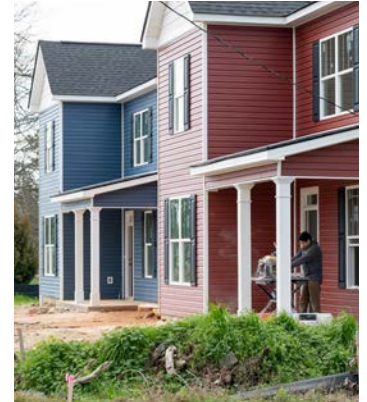
New Construction in Olde Town by Augusta Developer Wayne Millar.
